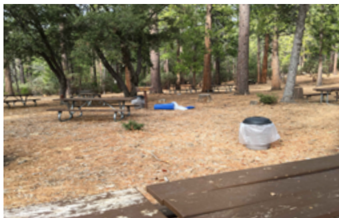
Walkway between parking and building has large gaps, excessive cross slope, and does not directly connect to the Designated Accessible Parking Space.
