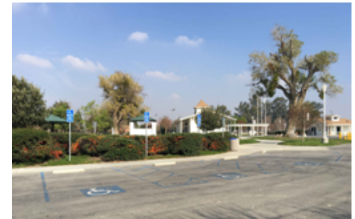
Striping, "No Parking" wording, and International Symbol of Accessibility are in need of repainting near the splash pad.
