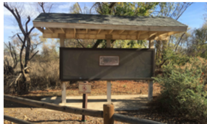
An informational message board is provided near the Day Use Area, but is not currently loaded with information readable from wheelchair level.
