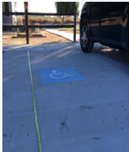
Parking space and access aisle exceeds 1:48 slope. Signage is not present. International Symbol of Accessibility is located deep within the space.
