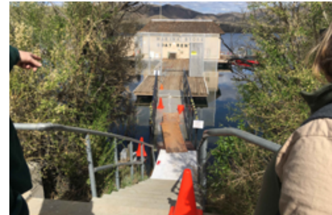
The only way to currently access the marina building is by stairs.
