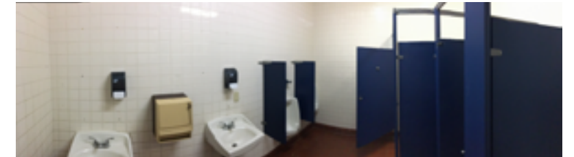
Panoramic view of men's restroom..
