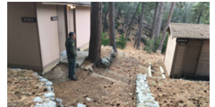
Exterior view of Restroom/ Showers
