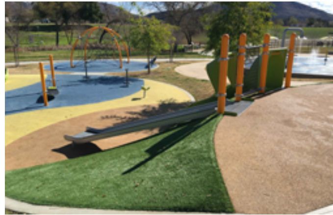
Play surface transitions to a steep incline with no provision for edge protection, to prevent wheelchairs from accidentally overtaking the top of slope.
