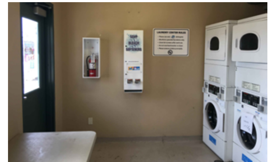
Laundry room interior view.
