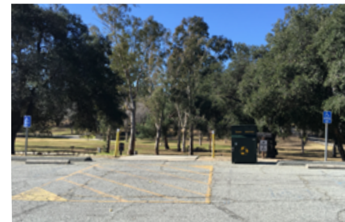
While signage was present at the DAPS within Meadow Parking Lot, most other accessibility components (striping, slope, loading zones) were severely deficient.
