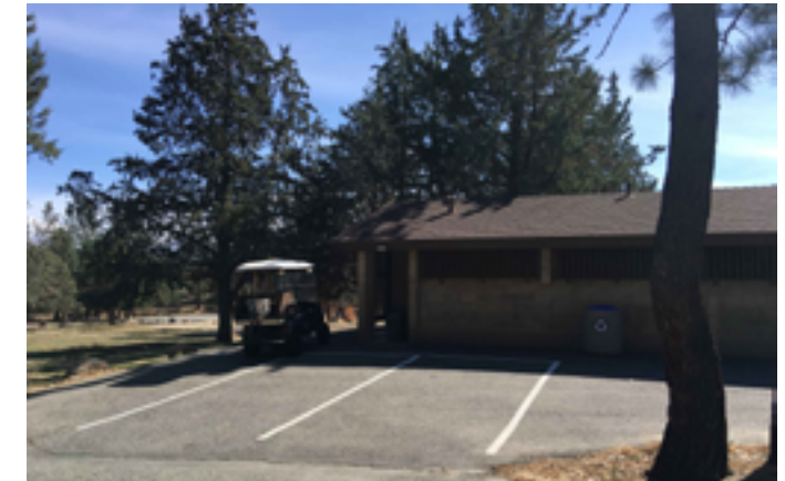
No Designated Accessible Parking is currently provided at the Indian Hill Restroom.
