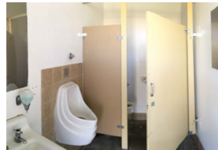
Interior view of restroom.
