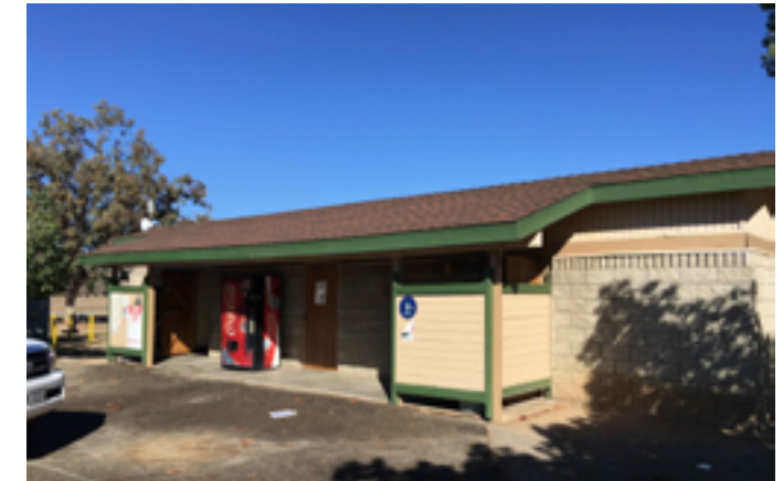
There is no Designated Accessible Parking Space within the parking lot near the Campground C Restroom.
