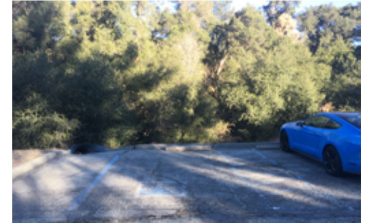
Typical condition of Designated Accessible Parking Spaces located throughout Bogart Park: deteriorated striping, missing or faded signage, excessive slope, etc. Pictured above: Pine Lot
