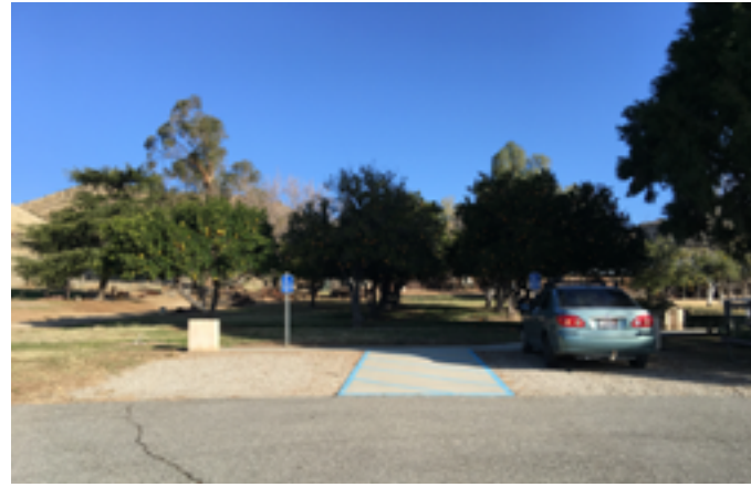
No van signage; no continuous smooth surface. No International Symbol of Accessibility.
