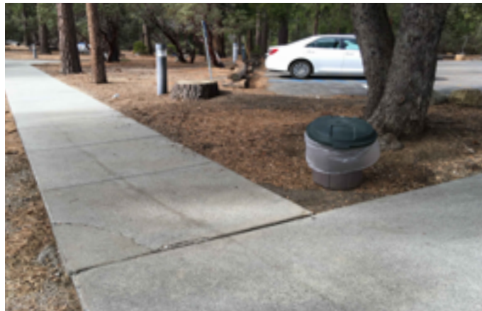
Walkway between parking and building has large gaps, excessive cross slope, and does not directly connect to the Designated Accessible Parking Space.
