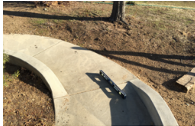
Narrow, steep turn in walkway connecting upper site features with Wagon Museum.
