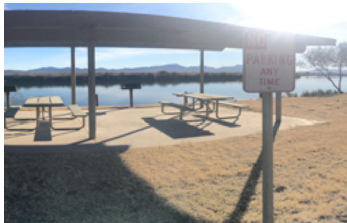
No accessible path is provided to any of the shelters from surrounding accessible park amenities.
