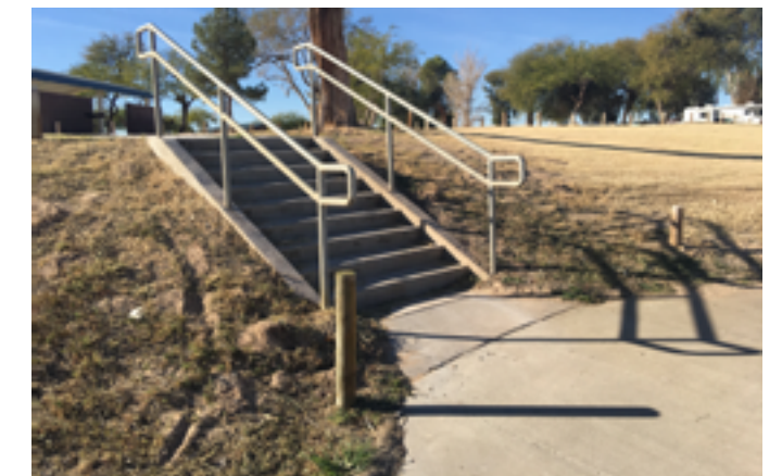
A staircase near the boat launch area has handrails that exceed 38".
