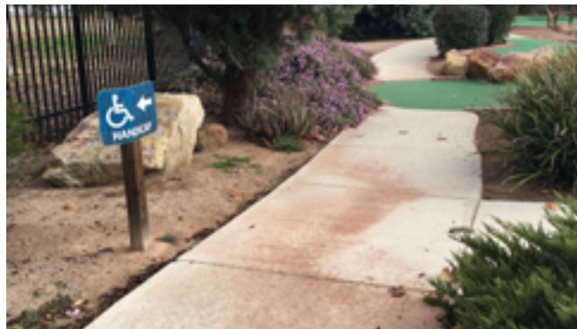
Replace signage to eliminate outdated "Handicap" terminology. The currently accepted term is "Accessible."
