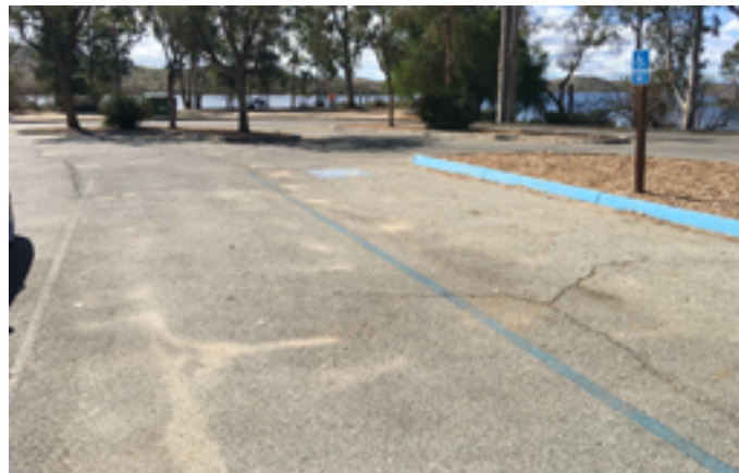
Provide an access aisle/ loading zone adjacent to Designated Accessible parking at Boat Launch areas.
