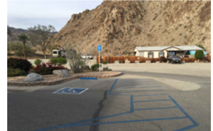
The Designated Accessible Parking Space near the Guard House at the Park entry is missing the “MINIMUM FINE $250” sign, and does not have detectable warning where the loading zone crosses into a hazardous vehicle area.
