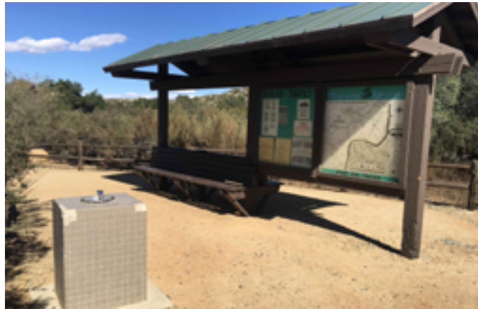
Drinking Fountain, Kiosk, and Benches within Parking Area: none of these provided amenities are compliant with current accessibility codes.
