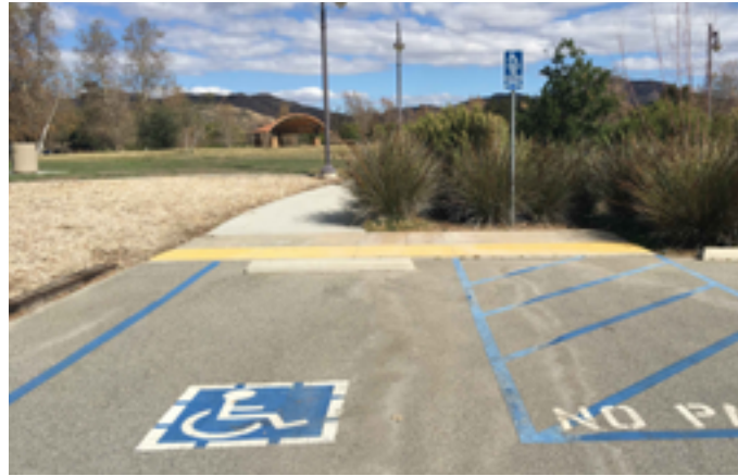
Signage, striping and detectable warnings were observed to be generally compliant within the most recently developed portions of the park.
