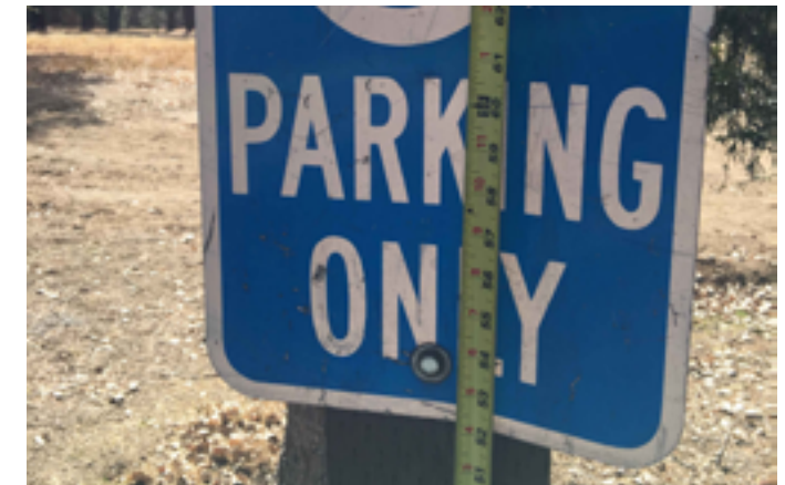
Signage shall be remounted with proper height clearance, as well as Van designation and "MINIMUM FINE $250" signage.
