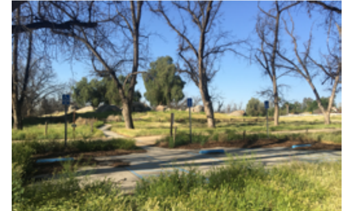
The site is currently overgrown, with vehicular access impeded to the parking area.
