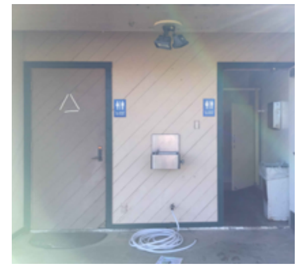
Exterior view of restroom entry.
