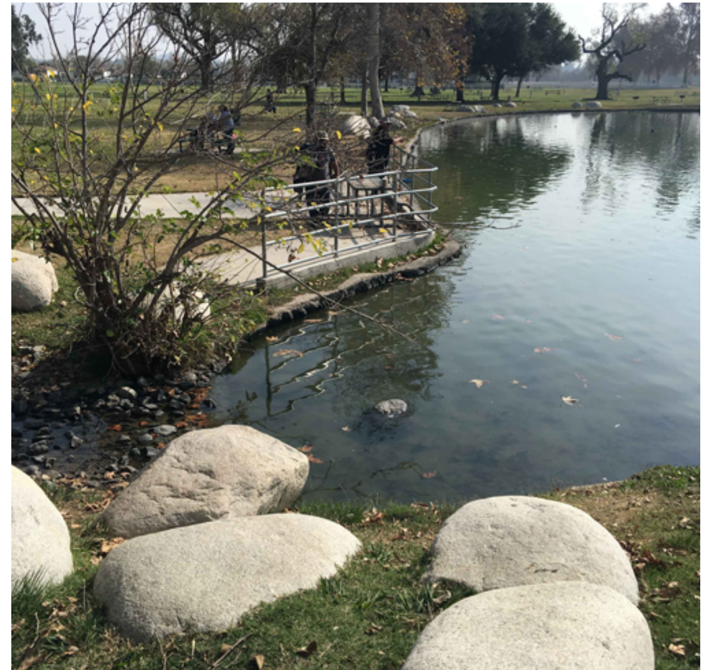
Modify guard rail to comply with the requirements of CBC 11B-1005.2.1, which states that at least 25 percent of the railings shall be 34 inches maximum above the ground surface.
