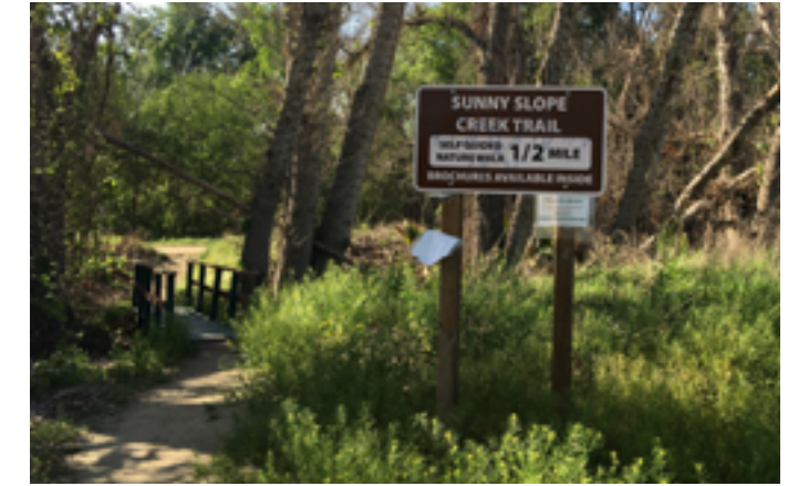
Access to the Sunny Slope Creek Trail requires users to cross a narrow footbridge with excessive cross slope and running slope, as well as lifted boards.
