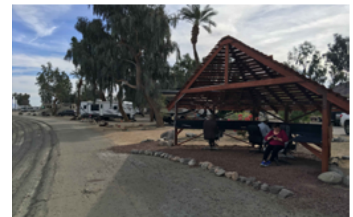
WiFi Hut within the RV portion of Lake Cahuilla does not currently provide an accessible path to the facility.
