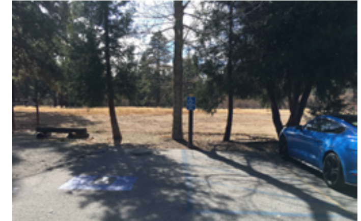
The sole Designated Accessible Parking Space is present on uneven asphalt with improper ISA markings, missing/ low signage, and has no accessible route between the loading zone and the adjacent restroom building.
