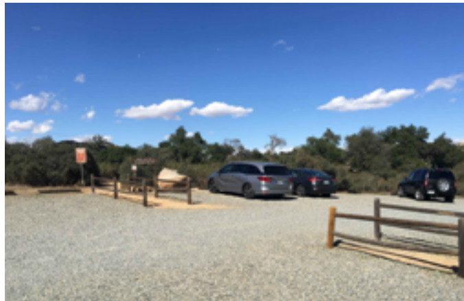
Gravel unmarked crossings do not allow for safe wheelchair or blind travel across the parking lot.
