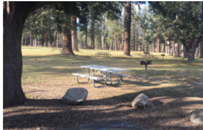
Excessive slope, debris on walkway surfaces, and subsiding asphalt all hinder the accessibility of the playground-adjacent parking.
