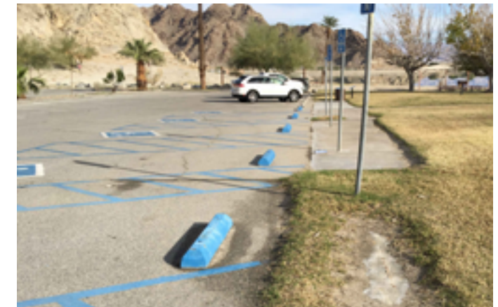
Designated Accessible Parking Spaces west of the Day Use area have a mix of compliant and non-compliant features. See action items.
