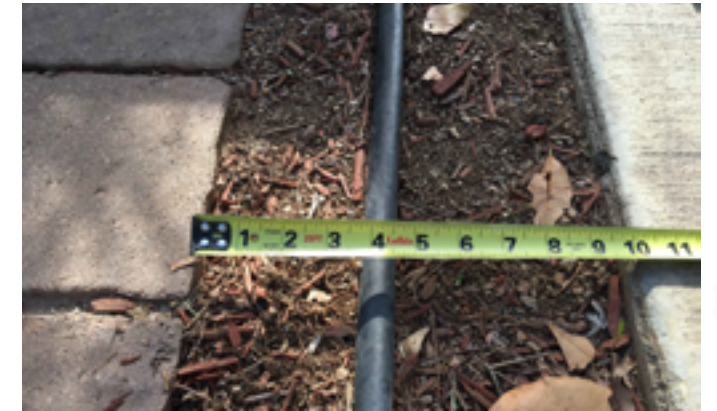
An irrigation dripline runs across a gap between paving materials at the entrance to the "Nature's Pathway" area, effectively preventing wheelchair access into the space.
