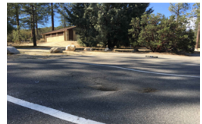
No Designated Accessible Parking is currently provided near Coyote Run Restroom.
