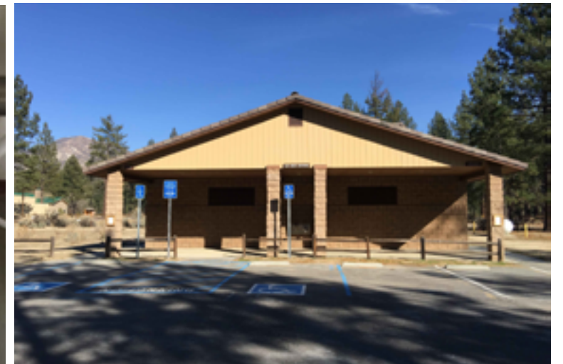
Restroom Entry from accessible parking
