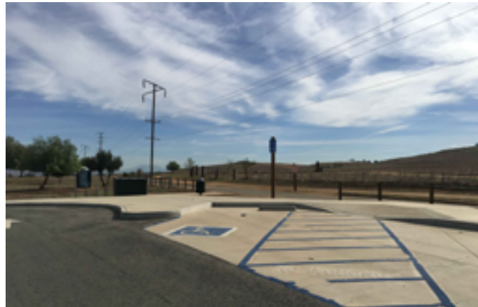
One Designated Accessible Parking space was provided with the applicable access aisle and curb ramp.
