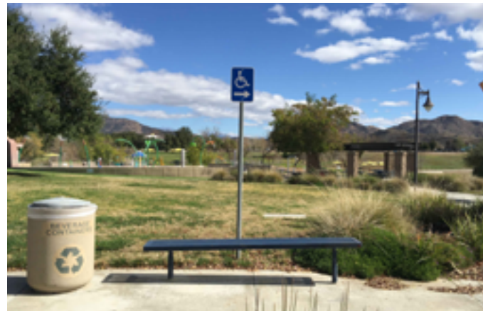
Replace benches with models providing back support, adjacent wheelchair companion seating, and mounted on a level surface so that the entire bench falls within the acceptable height range.
