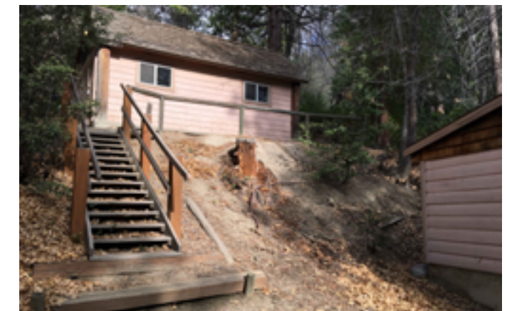
Cabins are set at varying pad elevations, requiring travel on steep stairs to reach.
