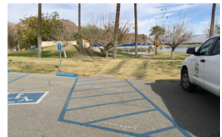
At the parking lot due south of the Day Use area, the loading zones do not connect to accessible routes heading to park amenities.
