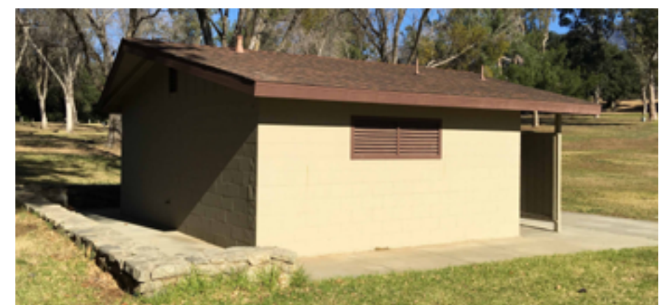
Back side of building.
