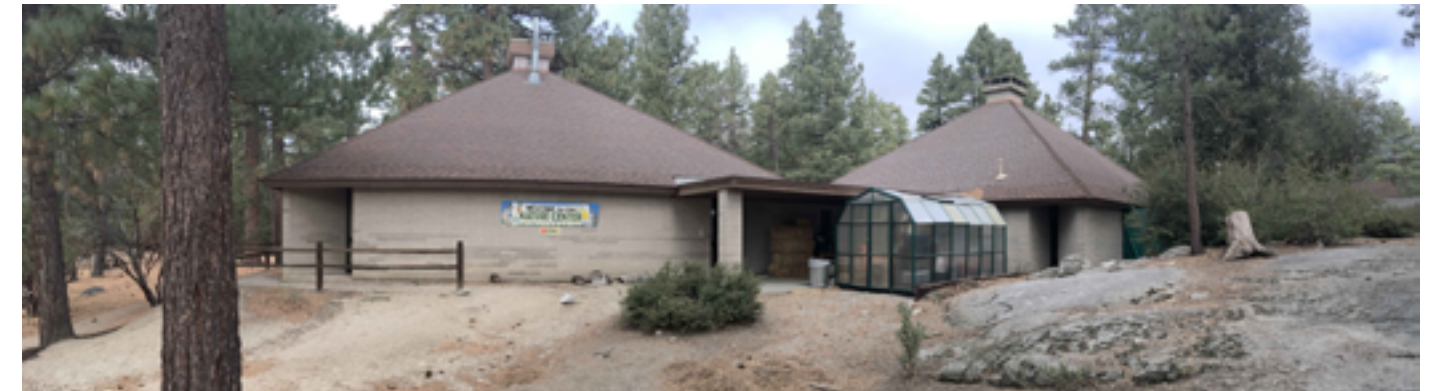
Exterior view of back of Nature Center building.
