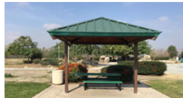
Wheelchair approach space clearances are not sufficient due to proximity of shelter posts.
