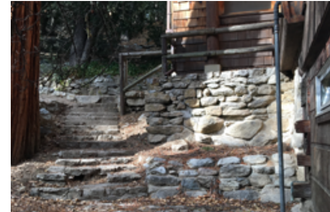
All existing structures are built into a steep hillside, and are only accessed by stone stairways, absent of handrails.
