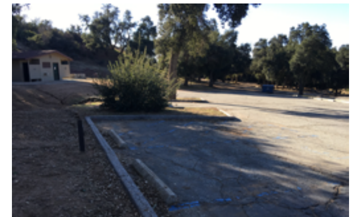
The DAPS within Manzanita Parking Lot also were observed to be severely out of compliance with current accessibility requirements.
