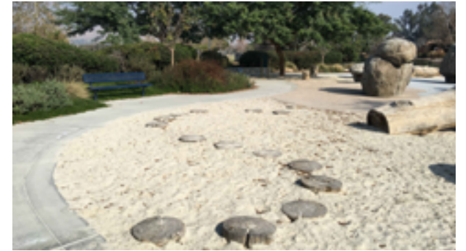
Wheelchair companion seating is not present next to provided benches at playground perimeter.
