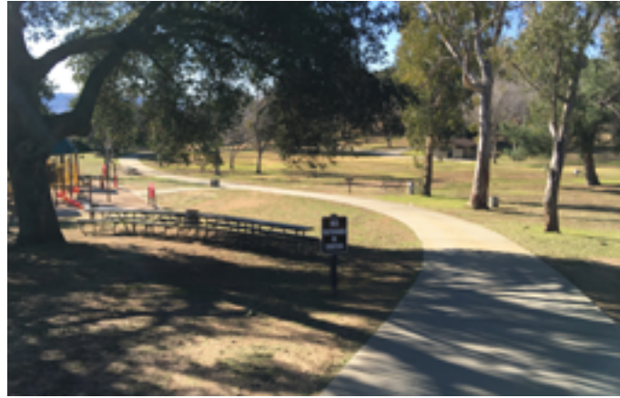
The majority of the Meadow concrete walkway exceeds maximum allowable slope requirements. There are also no picnic tables that meet the requirements of CBC 11B-246.5 and 11B-902.
