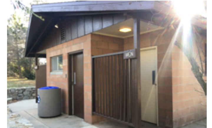
Exterior view of restroom.
