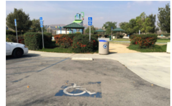
Faded ISA; no Detectable Warning at zero curb face.
