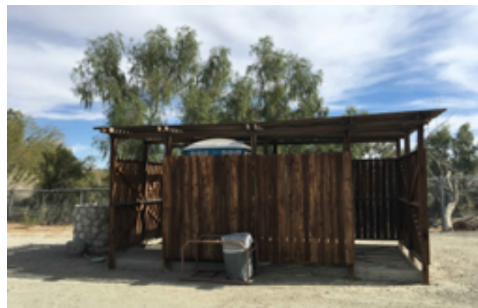
Typical example of portable restroom enclosure with no wheelchair-accessible portable toilet.
