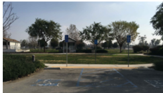
Concrete pad does not provide proper wheelchair approach clearances at accessible picnic table within campsite.
