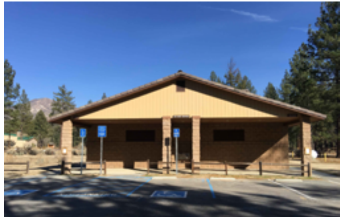
Designated Accessible Parking Spaces outside the New Group Restroom appear to be a fairly recent installation. These spaces are generally compliant, except the "MINIMUM FINE $250" sign is not present.
