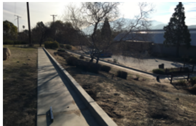
Long, narrow run with no landing or opportunity to pass; debris present on walkway surface; gaps present.
