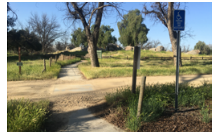
Minimum Fine signage not provided, nor are detectable warnings where the parking walkway enters the hazardous vehicular zone/ crossing.
