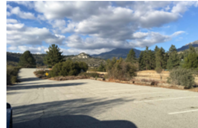
No DAPS are currently provided in the middle parking lot.
