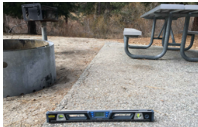
Amenities currently provided in the Designated Accessible Campsite are on an asphalt surface with excessive slope.
