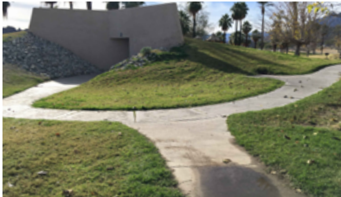
Steep, undulating walkway to restrooms. Standing water also present within walkway areas.
