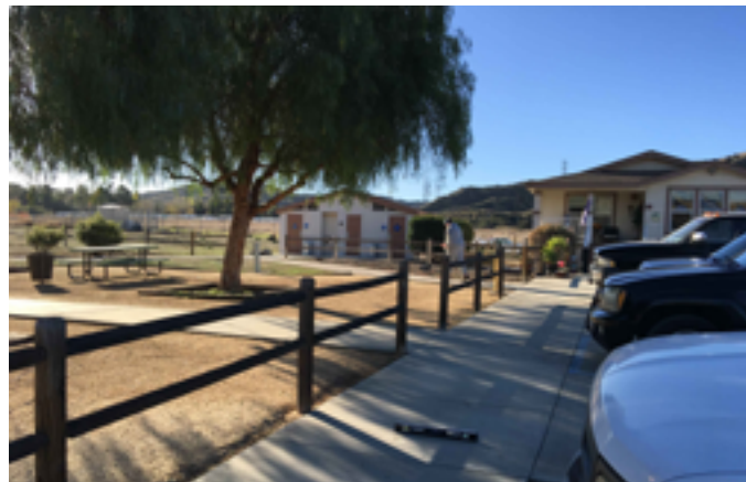
Designated Accessible Parking Spaces are located in close proximity to the ramped entrance to the schoolhouse and restroom building.
