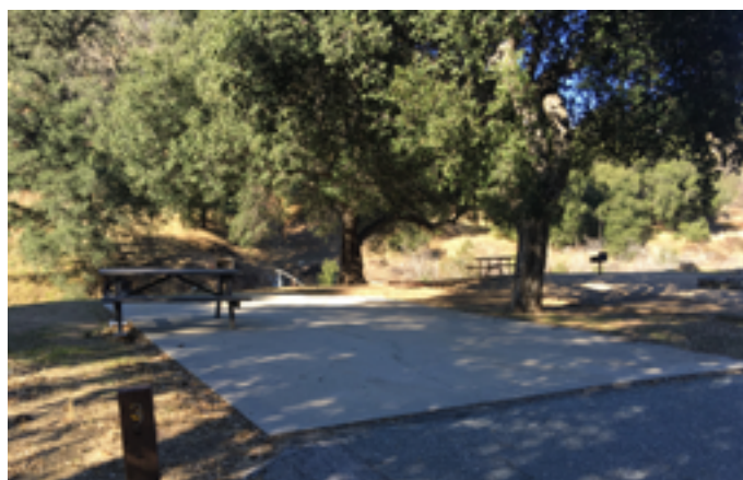
Campsite #3 is currently designated as the accessible site, but does not provide the required connection to sanitary facilities.
