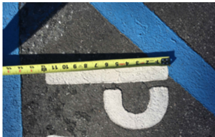
Pavement outside the New Group Restroom is currently in good shape; All painted stripes have good contrast. "NO PARKING" lettering is at proper size and location.
