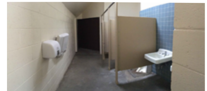
Interior of restroom building.
