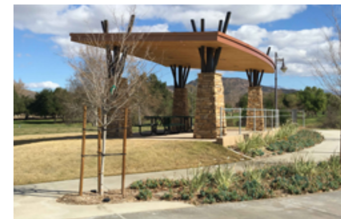
Where sloped walkway meets adjacent path, the turning space is somewhat ambiguous and potentially exceeds maximum allowable cross slope for wheelchair turning space.
