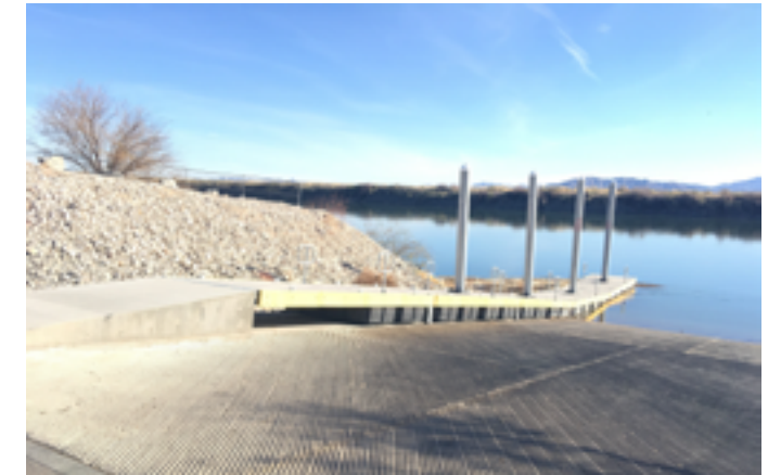
The boat launch exceeds the allowable slope for ramps, but meets the exception criteria listed in CBC 11B-1003. Due to topography constraints, signage should be provided to warn of the hazardous slope gradient.
