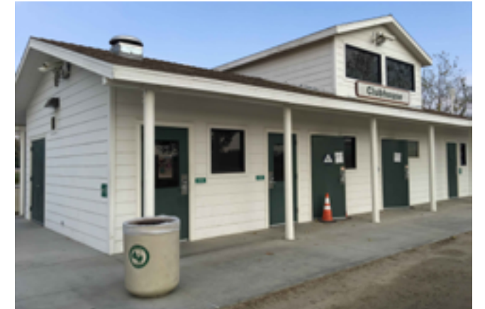
Restroom/ Shower exterior view.
