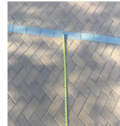
Loading zone/ access aisle striping is currently installed at over 4'; CBC requires 3' on-center, maximum.
