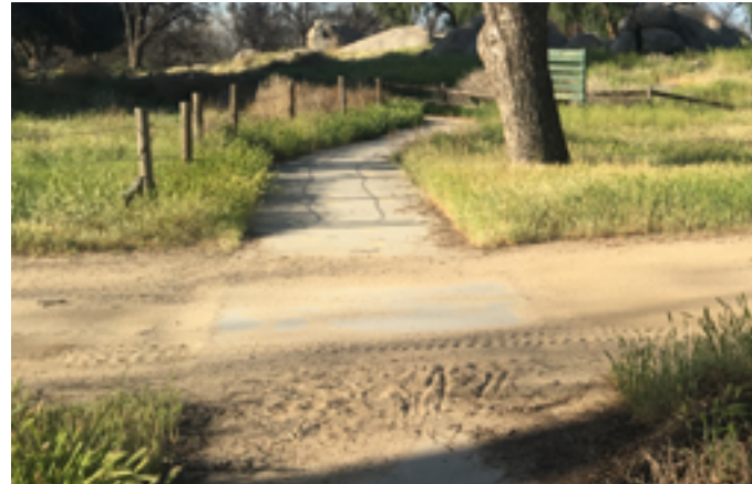
Truncated domes are not currently provided where the accessible walkway crosses the driveway.
