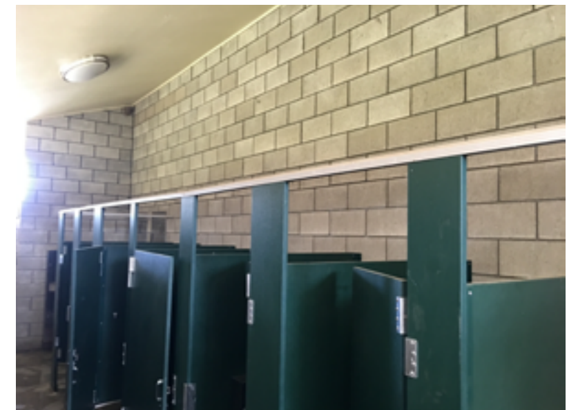
Interior view of building.
