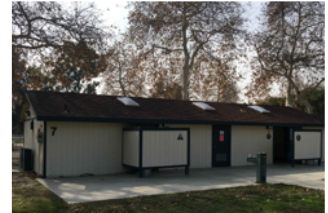
Restroom exterior view.
