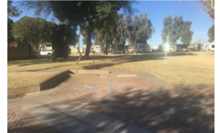
Despite the visually attractive qualities of this paver-set Designated Accessible Parking Space, there are several non-compliant attributes that need to be addressed.
