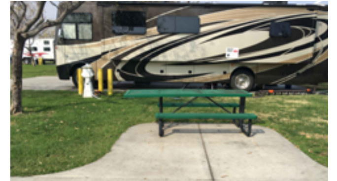
Concrete pad does not provide proper wheelchair approach clearances at accessible picnic table within campsite.
