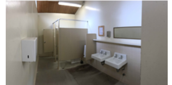
Interior view of Men's Restroom
