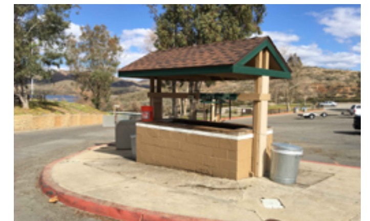
This fish cleaning station cannot be made accessible until the parking lot in which it is placed receives major renovations, likely including terracing.
