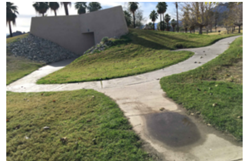
Non-accessible walks leading to restroom.
