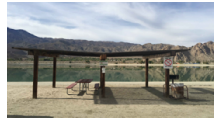
Example of one fishing shelter location with insufficient overhead clearance.
