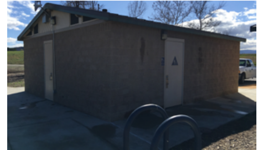
Exterior view of restroom.
