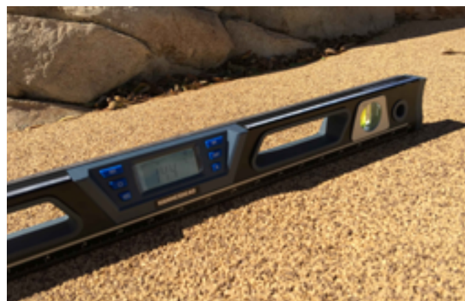
Another portion of play surfacing located parallel to an access ramp far exceeds allowable ramp slope.
