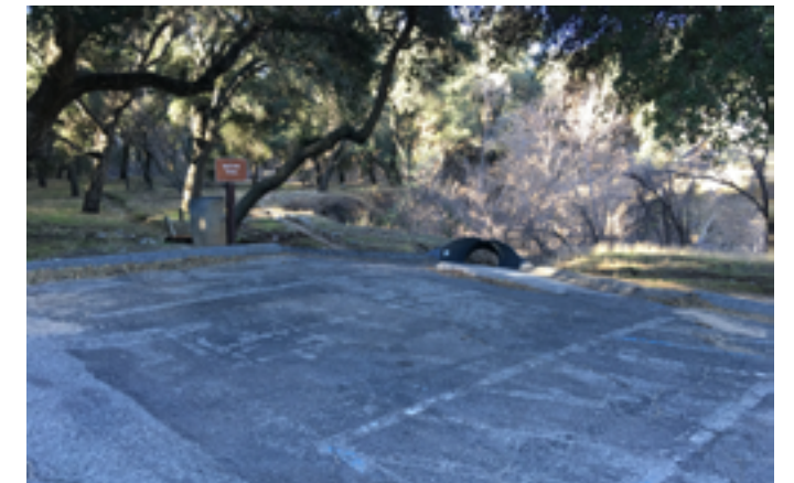
Existing DAPS at Oak Parking Lot. Signage is absent, markings are not clear. Loading zone does not connect to any accessible site amenities.
