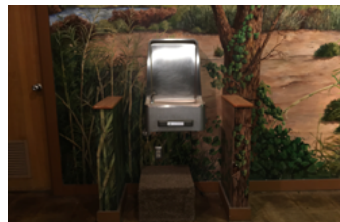
Drinking fountain missing its standing height counterpart.
