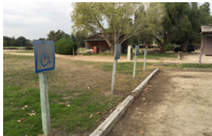
Designated Accessible Parking Spaces are currently by suggestion only, and are completely out of compliance in every way.
