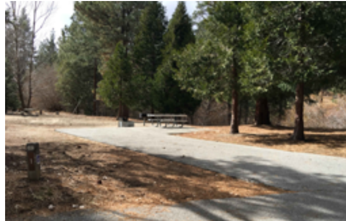
Campsite #1 is marked with an International Symbol of Accessibility, but does not provide an accessible route to the nearest sanitary facilities.
