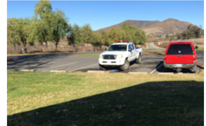
There is no Designated Accessible Parking Space within the parking lot near the Guard House.
