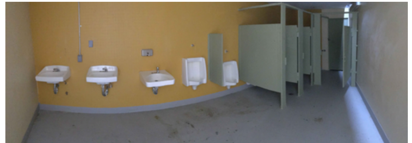
Panoramic view of inside men's restroom. Notable difference from previous restroom: no divider present between urinal and sink.
