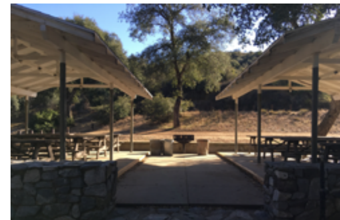
Steps between the shelters and barbecue area prevent accessible circulation.
