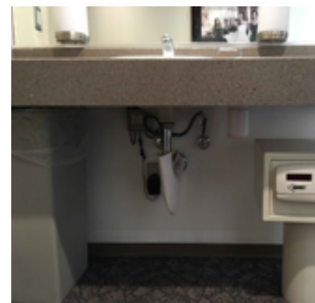
Waste container and property safe obstruct the wheelchair approach to the sink.
