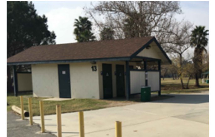
Restroom exterior view.
