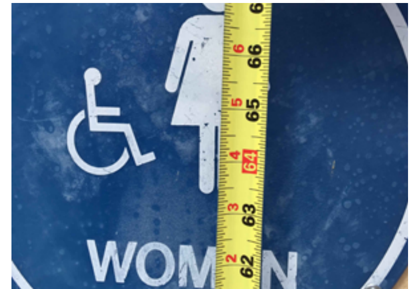
Geometric signage mounted too high.
