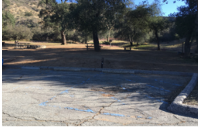
There is no accessible walkway connecting the Designated Accessible Parking Spaces with the Manzanita restroom nor to any of the picnic tables. Per CBC 11B-246.5, where picnic tables are provided, at least one picnic table, and one additional table for each 20 tables or fraction thereof, shall be accessible and comply with CBC 11B-902.
