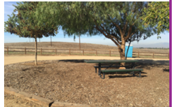
A picnic table and trash receptacle are provided near the park entrance, but are not on an accessible surface nor path.
