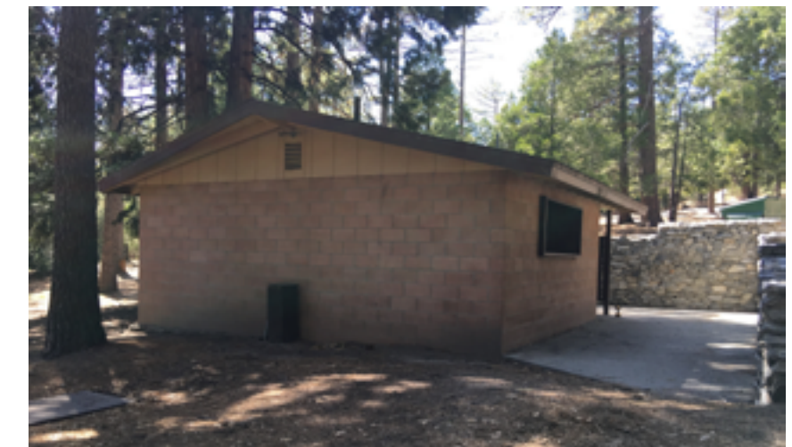
Rear view of restroom.
