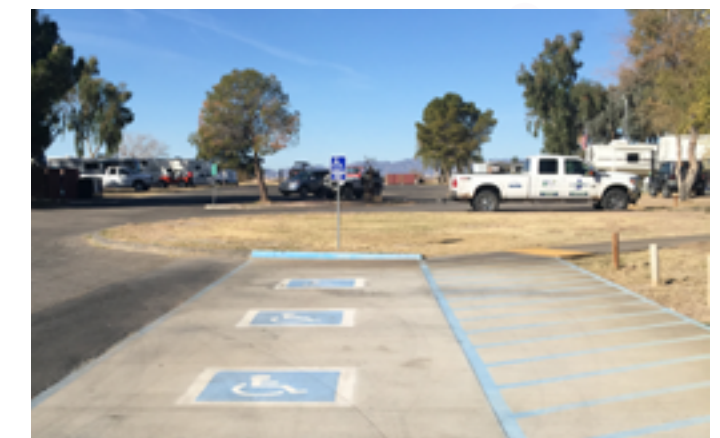
The "Boat Accessible" parking space needs to be renovated to meet the full requirements of CBC 11B-502.
