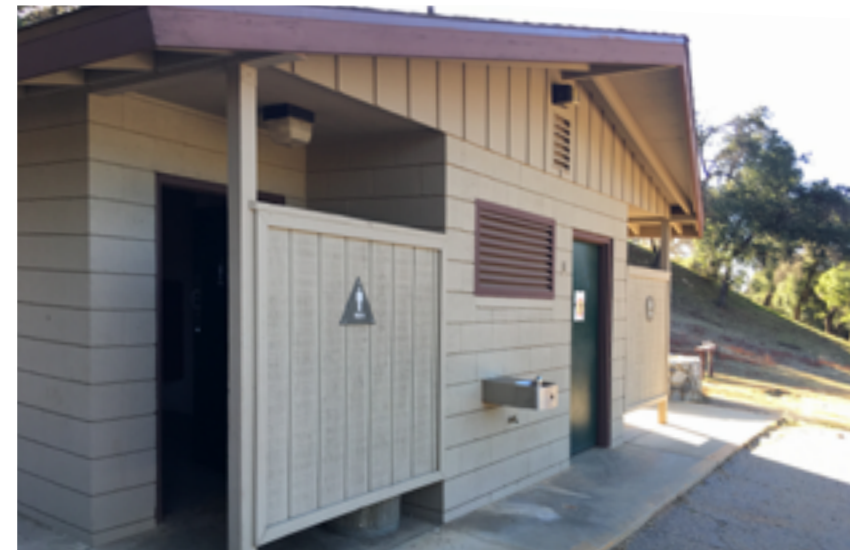
Drinking fountain does not have cane detection barriers from side approach, which are required if the fountain is not located within an alcove.
