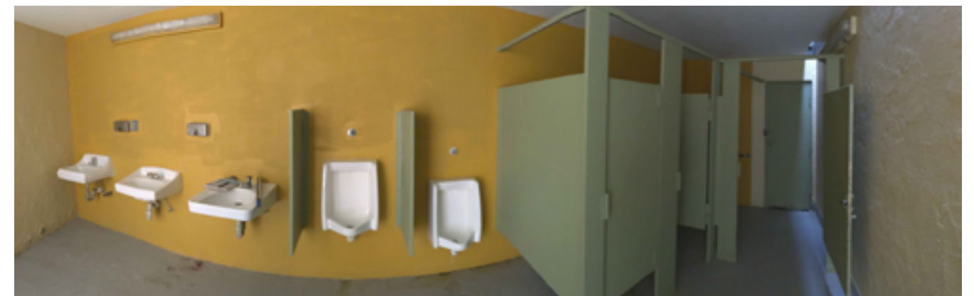
Panoramic view of inside men's restroom.
