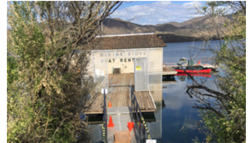
Marina and associated docks are completely wheelchair inaccessible.
