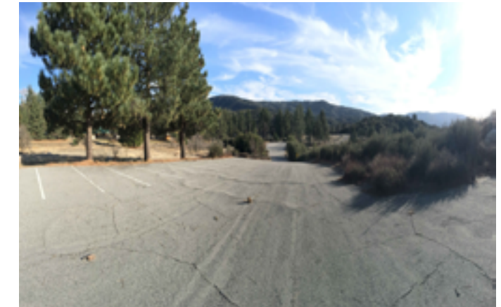
No DAPS are currently provided in the upper parking lot.
