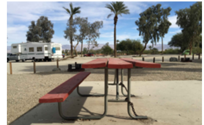
Existing picnic table within the Designated Accessible Campsite has a severely warped table top.
