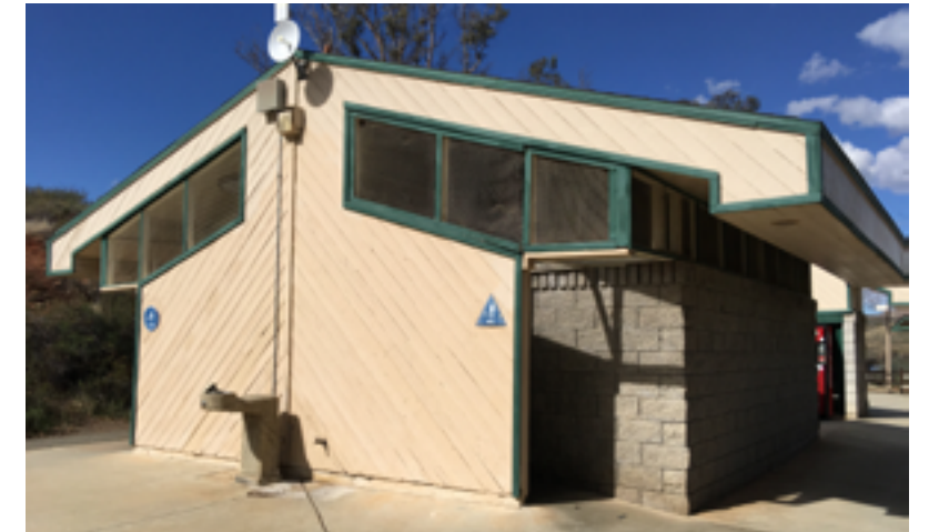
Exterior view of restroom.
