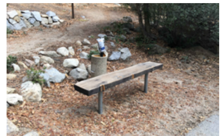
Existing benches do not provide the proper depth nor back support required by CBC 11B-903.
