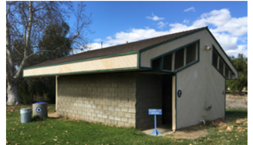
Exterior view of restroom.
