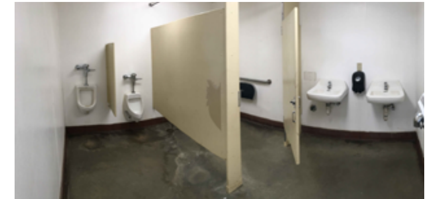
Restroom interior view.
