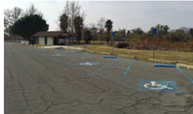
A variety of signage is provided near the Picnic Lakes restroom. Access aisles do not connect to accessible paths. "No Parking" designation is not present.
