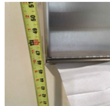
Paper Towel dispenser exceeds 40" AFF maximum at the towel exit point.
