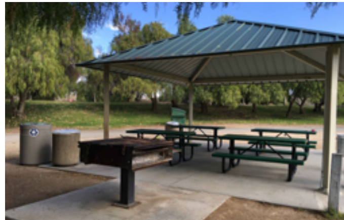
Group picnic shelter at Day Use Area #2 with no accessible path leading to it.
