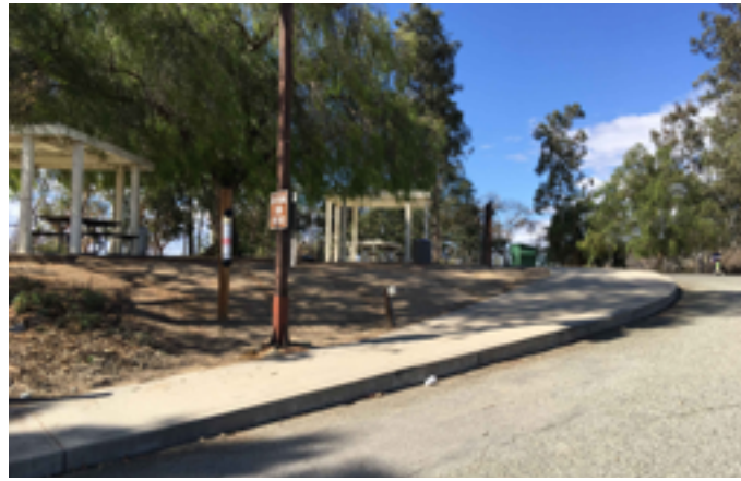
The walkway leading to the boat launch is in excess of allowable ramp steepness.
