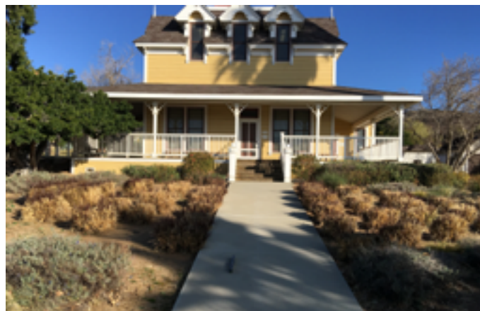
Very steep grade present at entry walk to historic house.
