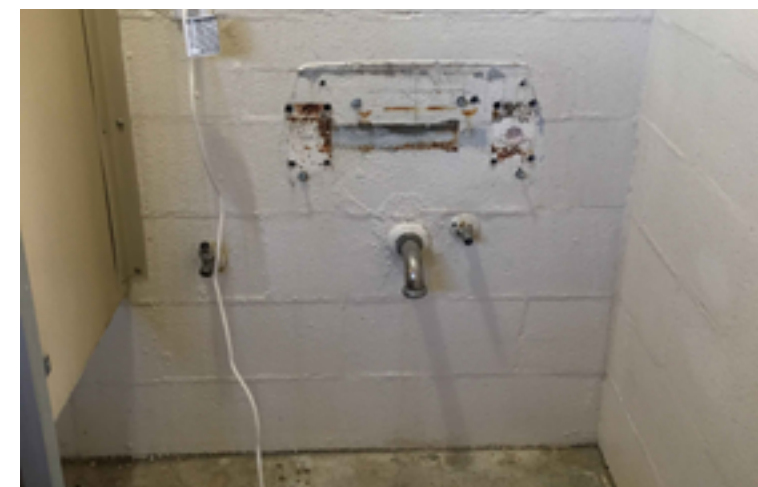
Renovations underway during inspection.
