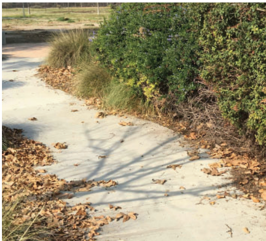
Above: Accessible walkway width compromised by leaf and plant litter at Rancho Jurupa Park.
